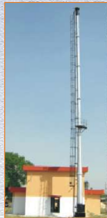
30 Mtr. high Chimney
